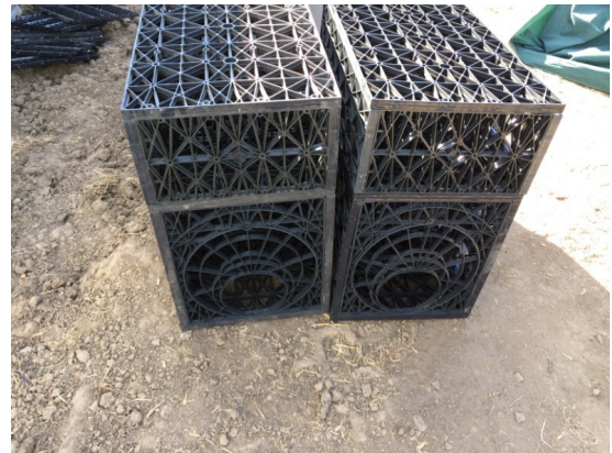
EcoRain Inspection/Cleanout Portal Tanks were installed.
