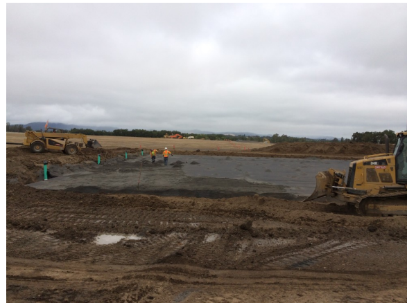
EcoRain Inspection/Cleanout Portal Tanks were installed.
